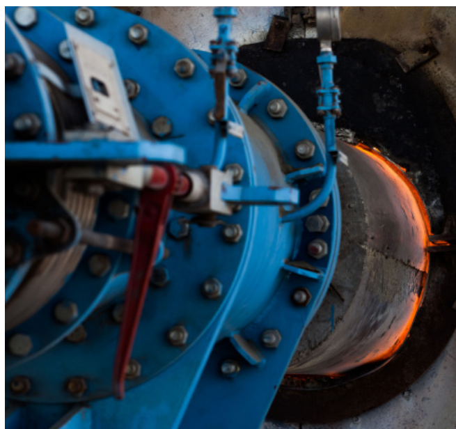
Rotary clinker cement kiln.
